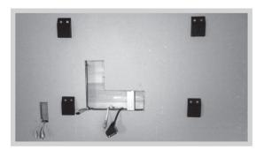
13. Fix all 4 LP brackets securely to the wall. Locate your cables in the cut holes/channels.
