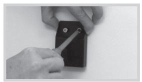
**12.** Screw the LP brackets in place using either a Phillips or 'posidrive' screwdriver. Tighten the screws until solid.
