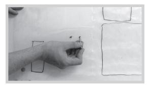
**8.** Using one of the screws provided, mark the screw holes, cable location and cutting/channelling guides through the template and follow up with the permanent marker.
