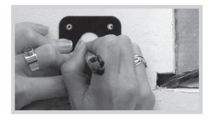
**10.** Place the ULP brackets over the marked screw holes and trace out the keyhole shape in the bracket using the permanent marker.
