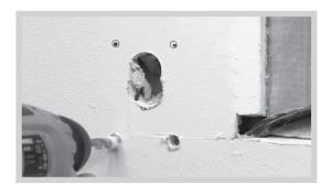
**11.** Drill as neccessary for width and depth of your bolt head to give a figure of eight shaped hole. Then, using a 6mm drill bit and using the markings as a guide, drill the screw holes on the wall no more than 50mm in depth.
