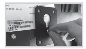
**4.** Sizing the bolt to the bracket. Loosen bolt off 2/3mm, place the bracket in desired keyhole slot and gently tighten. Remove bracket and repeat on other bolts. It must be tightened only enough for the bracket to be removed. Too tight and it will be difficult to fit, too loose and it will be shaky once fitted.
