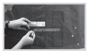
**3.** Using the permanent marker provided, draw around the cable ports (eg. SCART, HDMI, power, etc.). Ensure you do not mark these too neatly as you may require some room for movement later.
