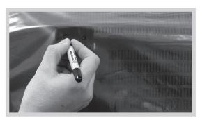
**6.** Drop the plastic template back down then mark out the screw holes on the ULP brackets with the permanent marker. If you find it useful then draw around the ULP brackets as well.
